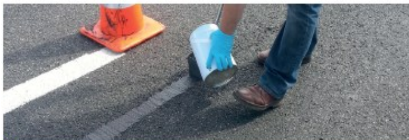
SAFETRACK CRACK INFILL APPLICATION
