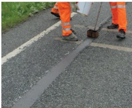
SAFETRACK INLAID ROAD REPAIR APPLICATION
